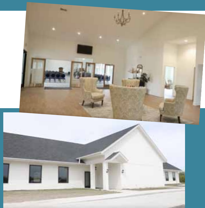
Stewards Foundation provided a loan as well as construction administration advice in assisting Lake Country Bible Chapel with the construction of their new facility
